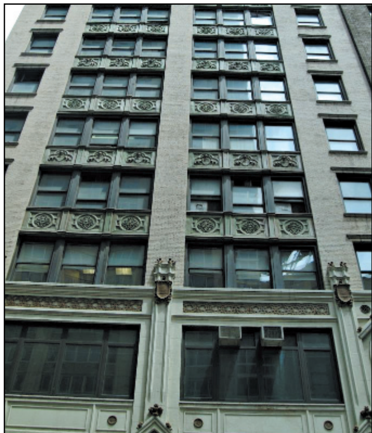
Perfetto represented an individual investor in a 1031 exchange transaction involving this W. 38th St. building. Marshall Cohen, Matia Nikolovienis and Christine Mulryan, all from Cohen & Perfetto, also worked on the project.
